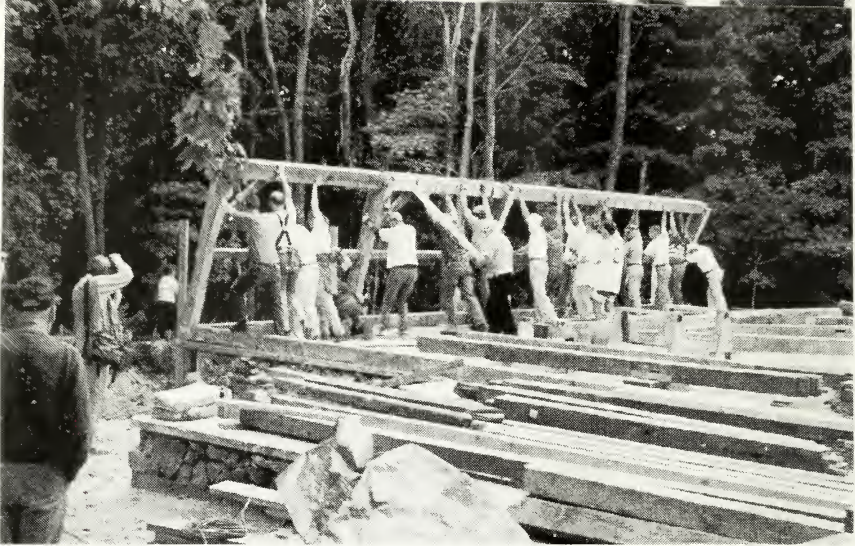
Raising of the rear shed wall by volunteers
